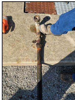
Diffuser replacements
