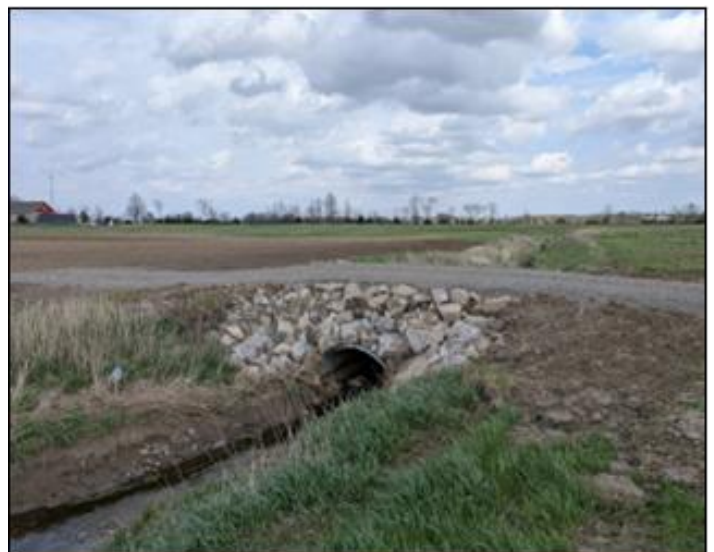
A corrugated metal pipe culvert to allow a field road to pass over a drainage ditch
