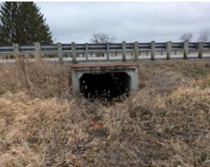
A concrete box culvert to allow Willis Ditch to flow under State Route 347 in Union County, Ohio
