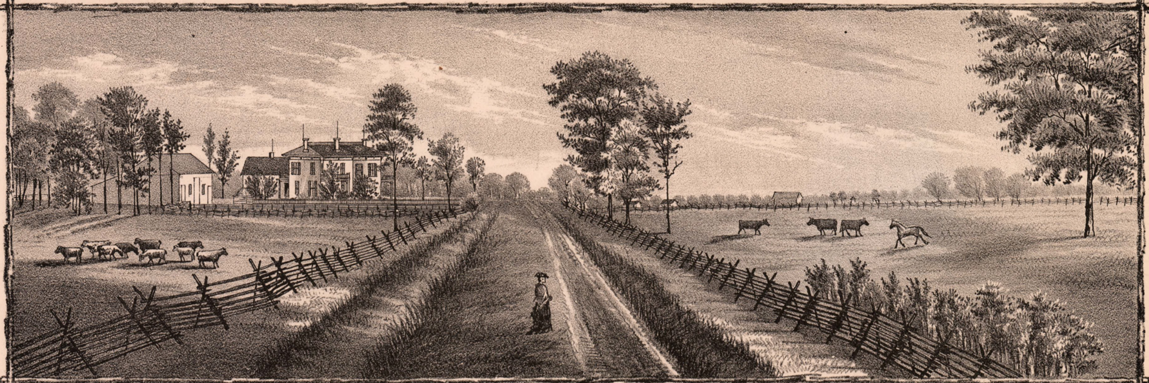
VIEW FROM THE WEST.
