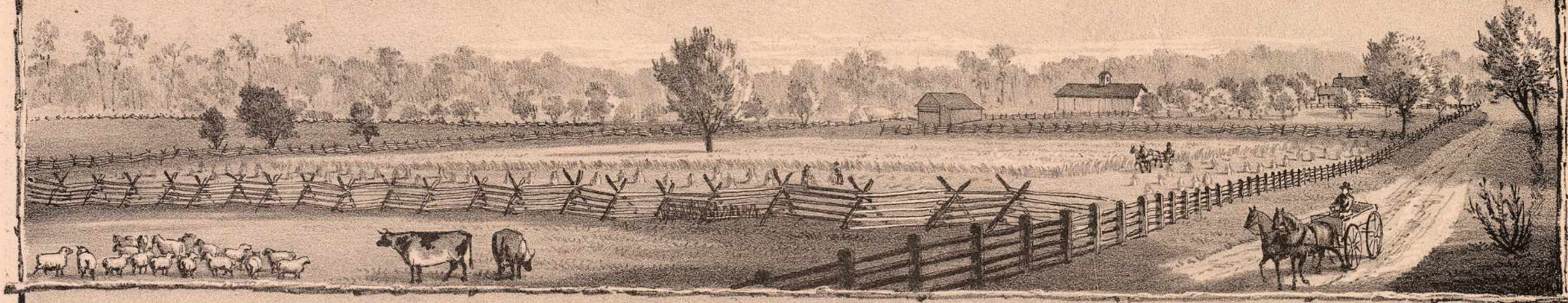
FARM VIEW FROM THE NORTH WEST.
