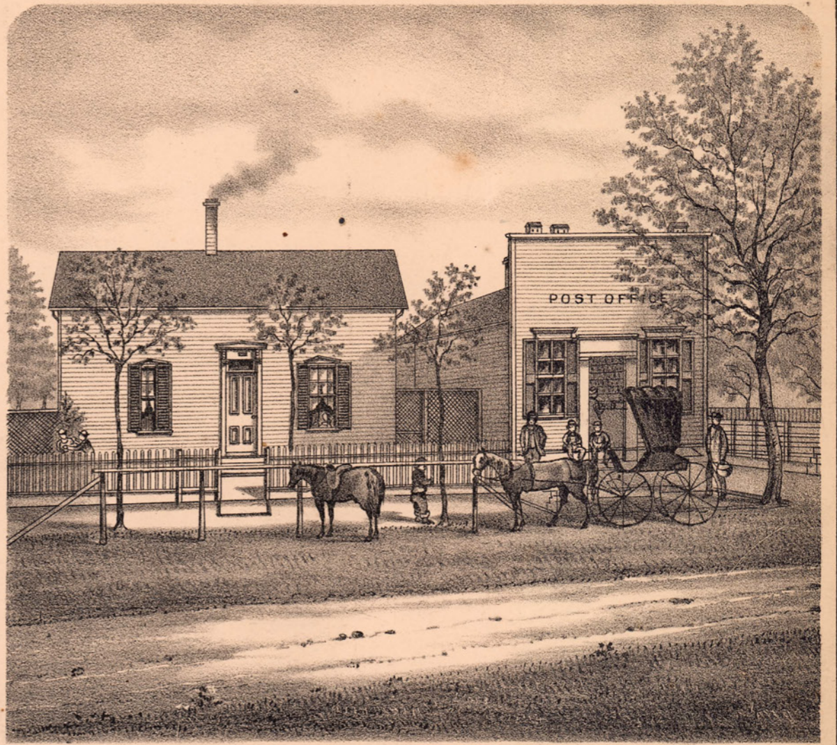
STORE AND RES. OF OTHO HARDMAN, ROSEDALE, PIKE TP. MADISON CO. OHIO.
